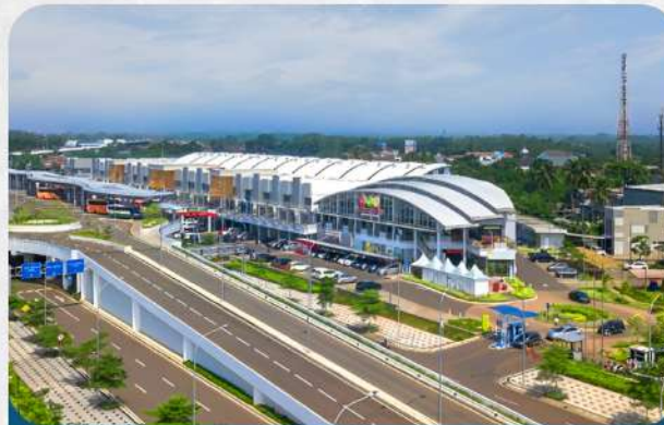
Terminal Intermoda BSD
